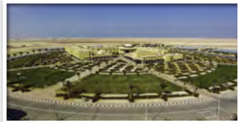
RAS LAFFAN EMERGENCY & SAFETY COLLEGE - QATAR -7.7mtrs
