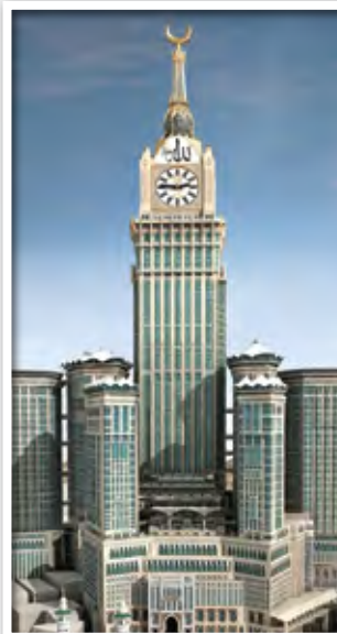
DOKAEE TOWER -H PLAZA - SAUDI ARABIA - 5mtrs
