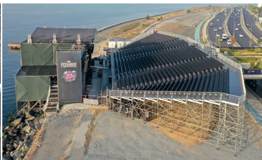
Stage and stand made of standard Allround components and Event System
